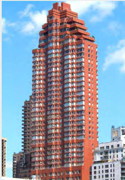
THE BELAIRE CONDOMINIUM 524 East 72nd Street, Manhattan 134 apartments
